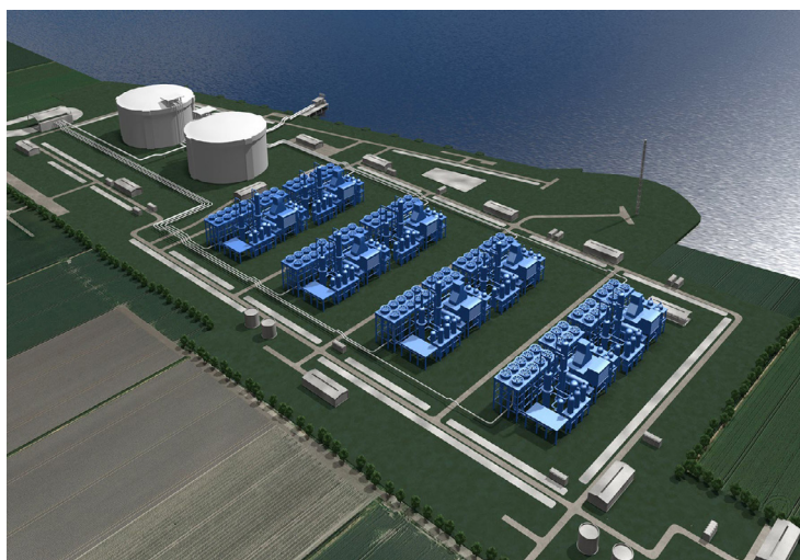
Figure 1. 3D representation of contemporary mid scale multi-train LNG production and export plant.
